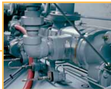
The ST799GCDP03R31 starter is piped for use with gas on a Waukesha F3521GU used for power generation.
