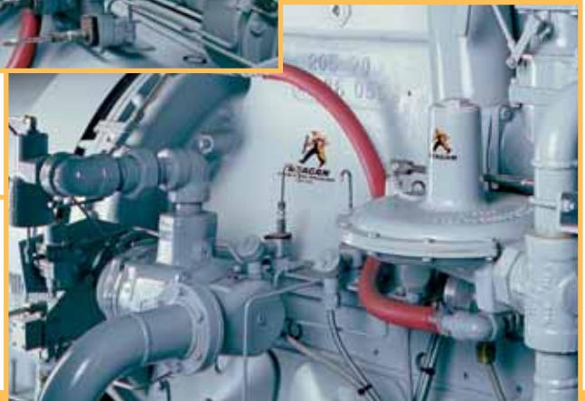
The ST799GCDP03R31 starter is piped for use with gas on a Waukesha F3521GU used for power generation.
